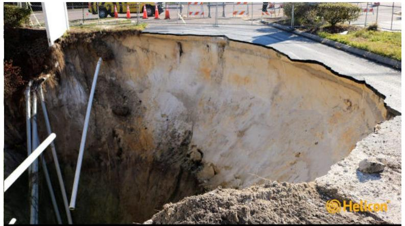
Fill the voids, cracks, fractures, and cavities while stabilizing the granular material and improving the physical properties of the soil and limestone.
