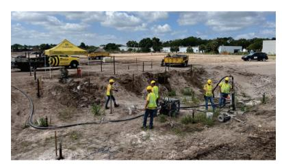
Compaction grout pumped into 56 injection points per the soils reports findings. 7,896 lineal feet of drilling and 1,344 cubic yards of concrete.
